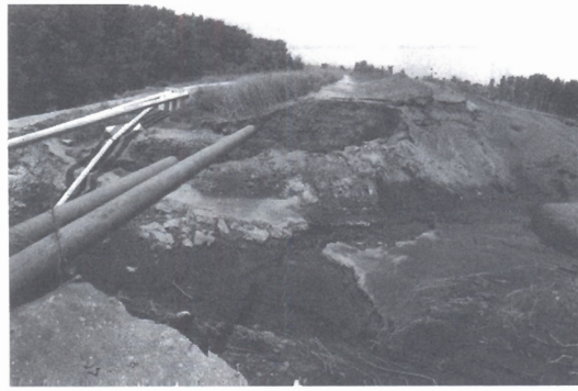
Figure 1. Dike-break site (breach opening).
