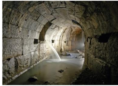
Figure 3. Ancient Rome's main sewer line, the Cloaca Maxima. Still used for street run-off, the sewer's entrance, ancient stone inlet, can be seen from Ponte Palatino (after Lamprecht).
