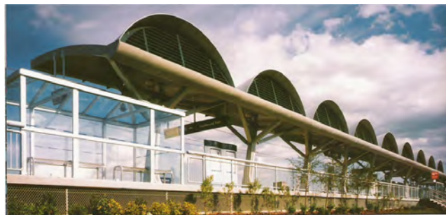
Figure 12. Shawnessy railway station, Canada (2004) – the thinnest concrete shell ever constructed (UHPRC shell, 6 m × 5.15 m in layout, thickness 18 mm, 150/25 MPa UHPRC compressive/tensile strength)
