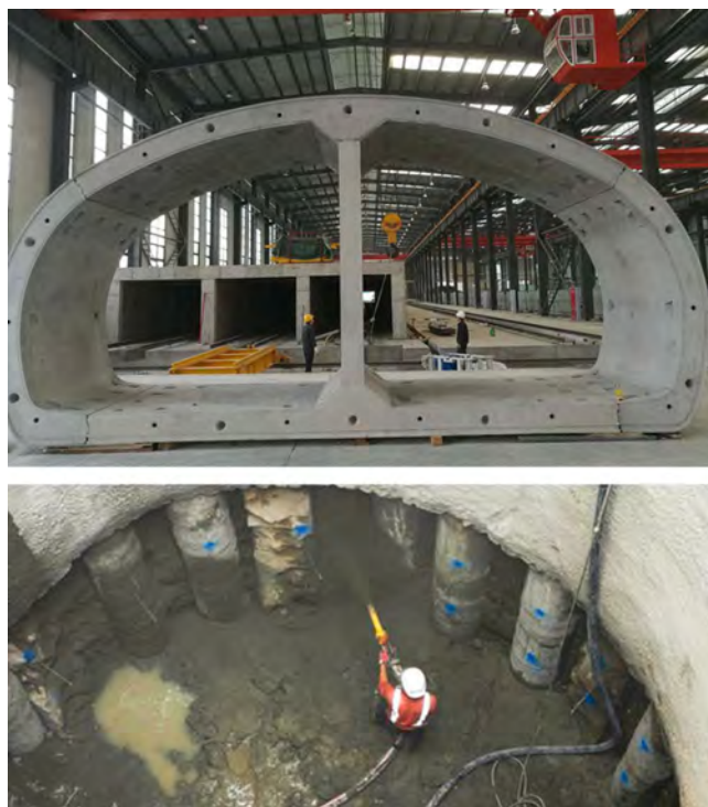
Figure 8. FRC precast tunnel lining segments (up) and FR shotcrete in underground structure (down)
