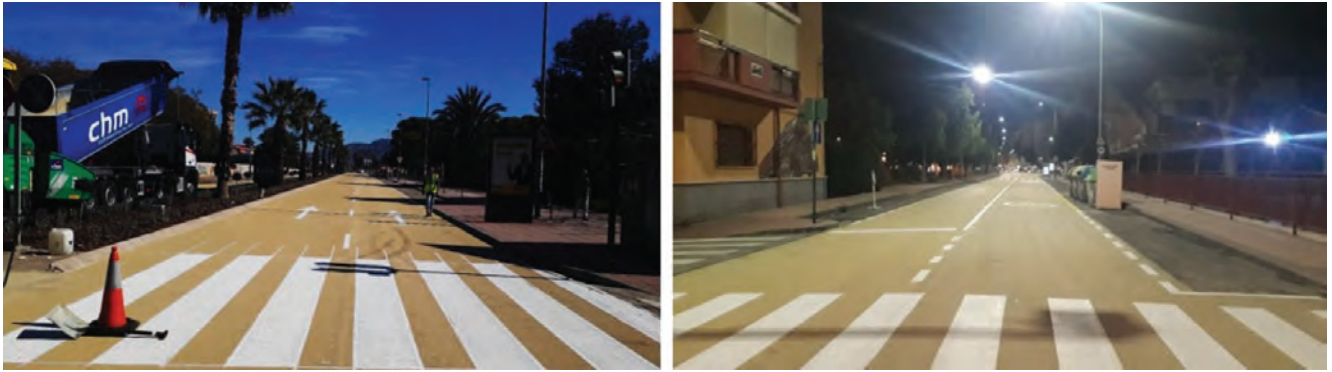
Figure 11. Cool pavement just after its installation in two different streets and in different light conditions: day (left) and night (right)
