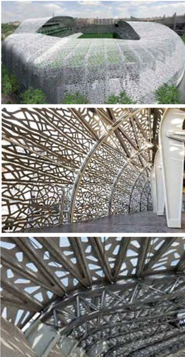
Figure 13. Jean Bouin Stadium, France (2013) – roof and façade self-supporting lattice Ductal® UHPC panels (roof panels 8/9 \times 2/2.5 m, thickness 3.5/4.5 cm, façade panels 9 \times 2.5 m, thickness 11cm)
