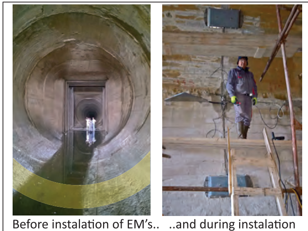
Figure 20. F-B tunnel, inlet cross section F-B IN before installation of equipment (left) and during the installation (right)
