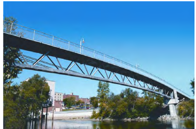
Figure 11. Sherbrooke pedestrian bridge in Canada (1997) – span 60 m, precast prestressed RPC (200 MPa)
