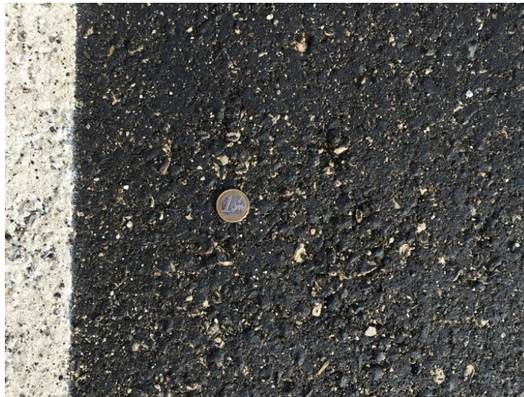
Figure 8. 100% cold recycled binder layer in Spain after completing the compaction
