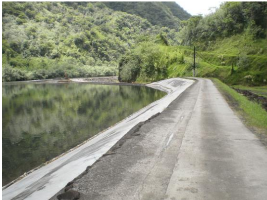
Pogled sa brane ka prelivu View from dam to spillway
