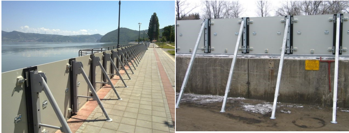
Slika 4. Predložena mobilna oprema Figure 4. Proposed mobile protection
