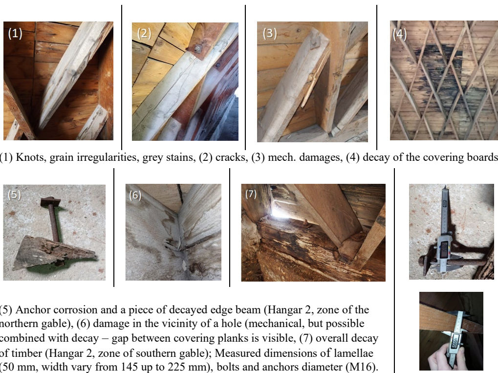
Figure 8. Observed damage types (brief overview) and measured dimensions [2]
