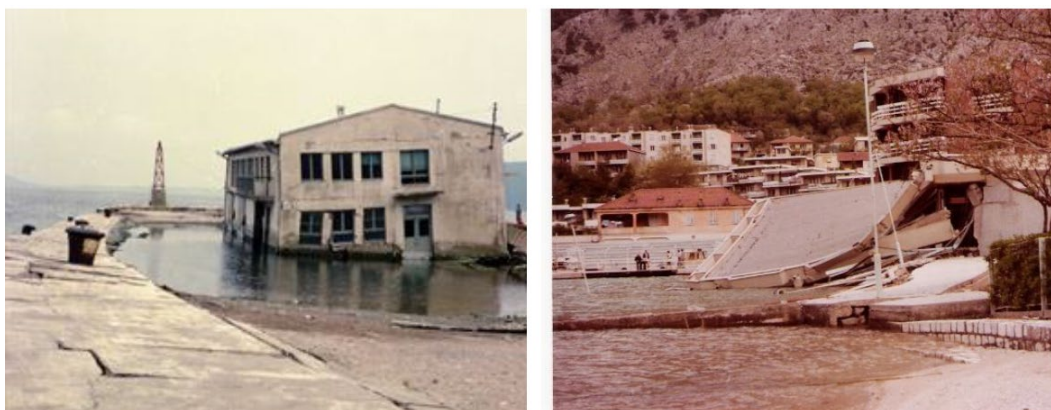
Figure 2. Subsidence of the terrain under the warehouse in the port of Zelenika, left picture; Heavy damage to Hotel Fjord – Kotor city, right picture
