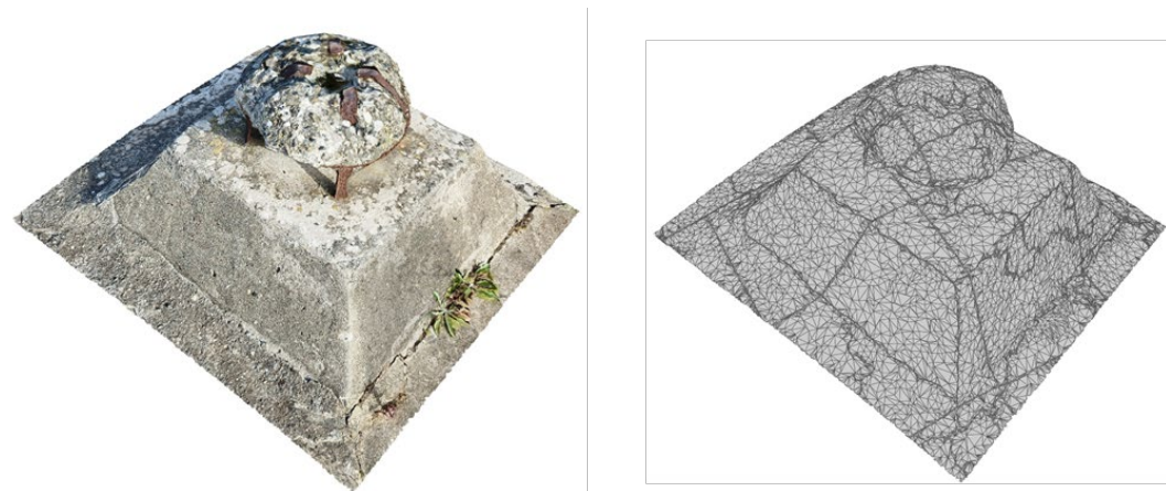
Figure 11. Representation of a poorly preserved vent. Left: realistic version, Right: point correlation version.
