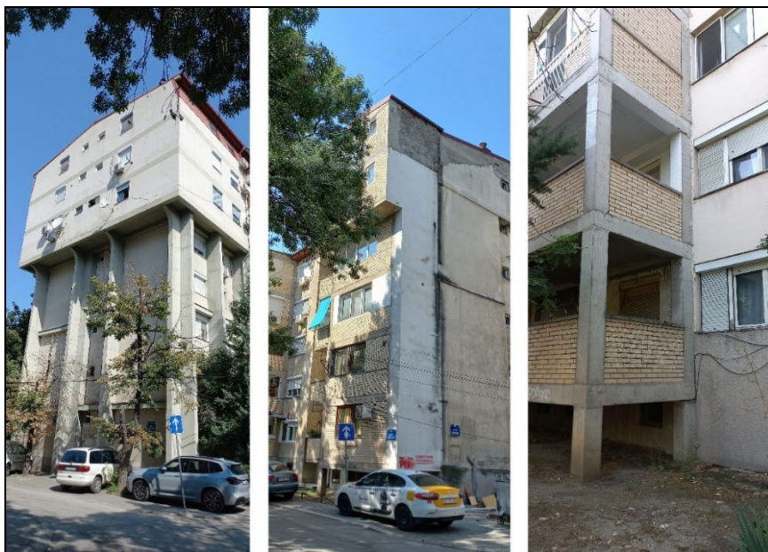
Figure 6. Buildings with mixed structure with use of expansion joints. Source: photos by K. Edip.
