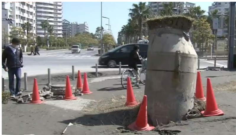
Figure 3. Sewage manhole that broke out on the surface due to the liquefaction, Abiko city in Japan
