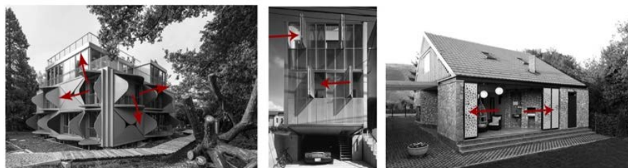
Figure 5: The principle of opening and closing, Ballet house, Tokio Steel house, House in Smilovci
