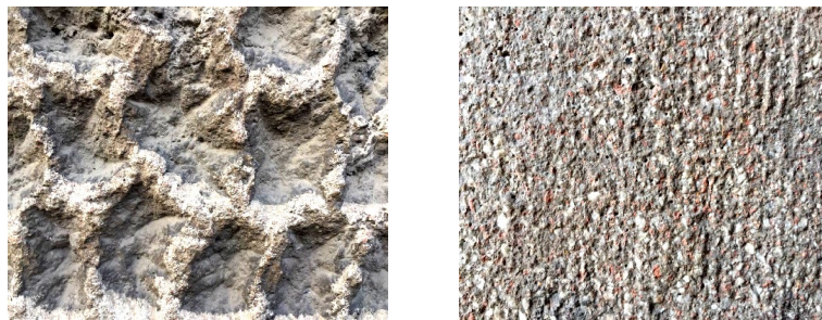
Figure 3: Various types of decorative picked/carved façade (Author of the photos: arch. Mirjana Devetakovic Radojevic, Ph.D.)
