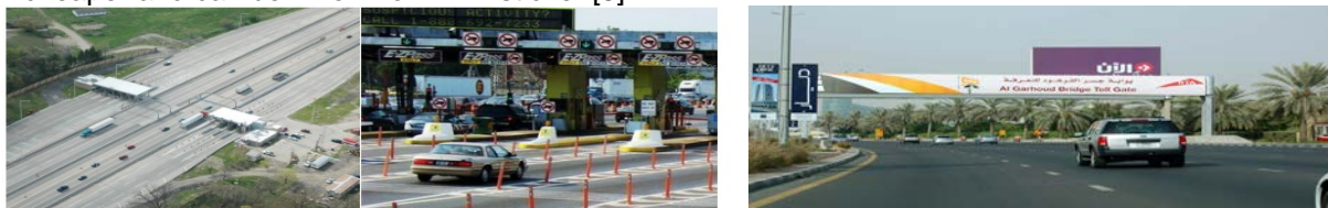
Figure 8. RFID ETC with and without barriers tolling
