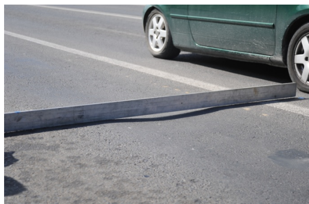
Figure 15. Deep ruts near the traffic lights Source: (custom measurements)
