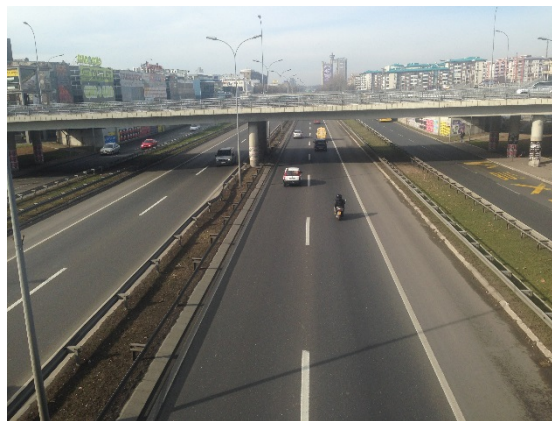
Figure 10. E75 pavement condition in 2016
