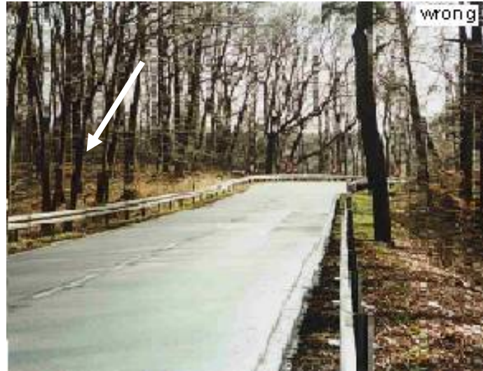
Figure 17. Three oversized chevron signs are not visible against the background in an accident curve [5]
