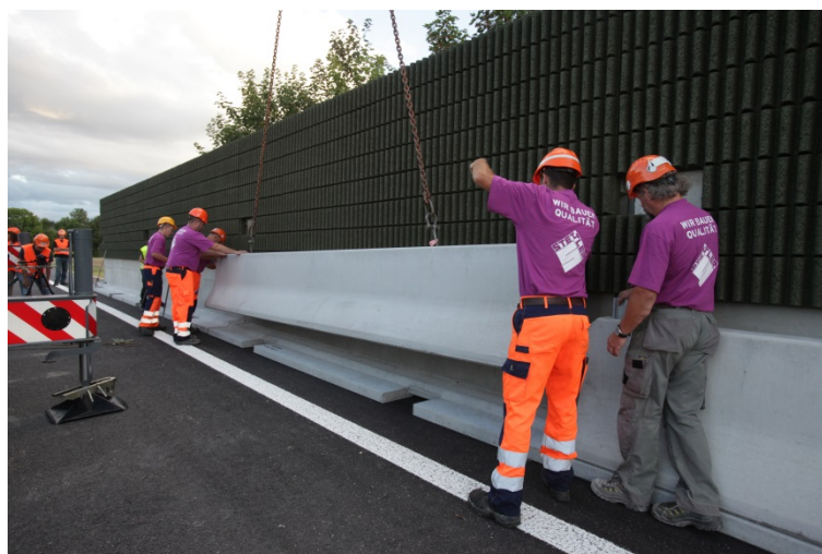
Figure 14. Installation of DB 80 LSW-R, Switzerland Source: Photograph © DELTA BLOC International GmbH
