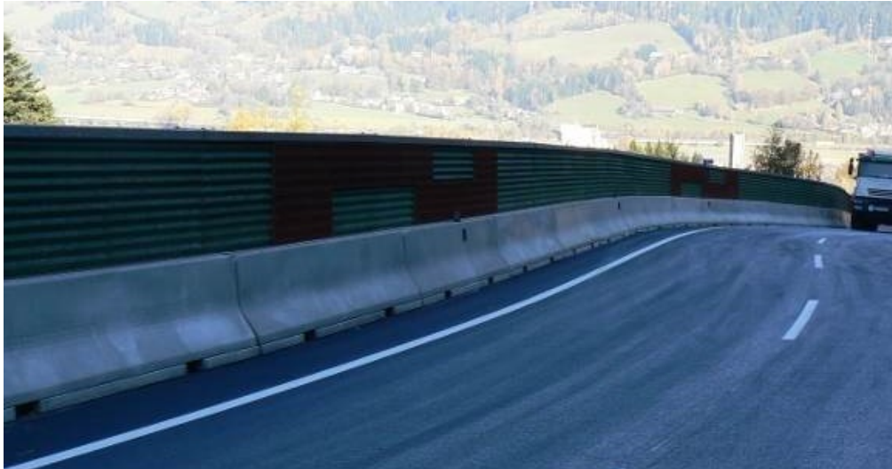
Figure 4. The noise barrier was sufficient with a height of only 2m because of the proximity to the noise source Photograph by © DELTA BLOC International GmbH
