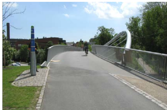
Figure 10. Destabilisation by a non-orthogonal and unsymmetrical suspension: balance is disturbed and field-depended users tend to swerve to the right [17]
