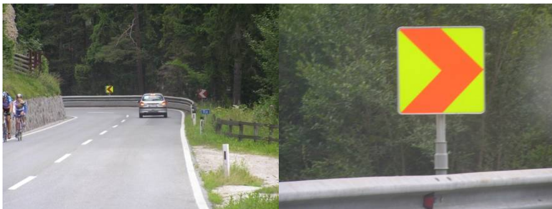
Figure 18. Improved visibility of signs by use of yellow background instead of red (source: photo from Austria, Hans-Joachim Vollpracht, 2008)
