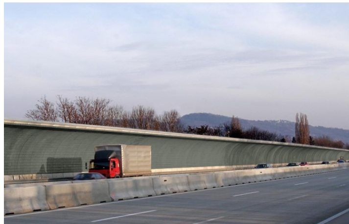
Figure 11. Example of an arched noise barrier wall, Austria Source: Photograph © Ralf Dimberger DELTA BLOC International GmbH
