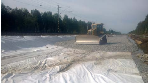
Figure 1. Photo from Riippa-Eskola railway construction project.
