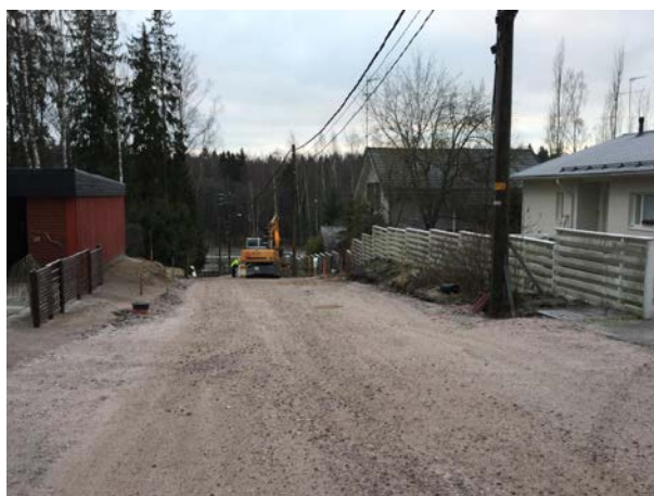
Figure 2. Street renovation site (Tammitie, Espoo).
