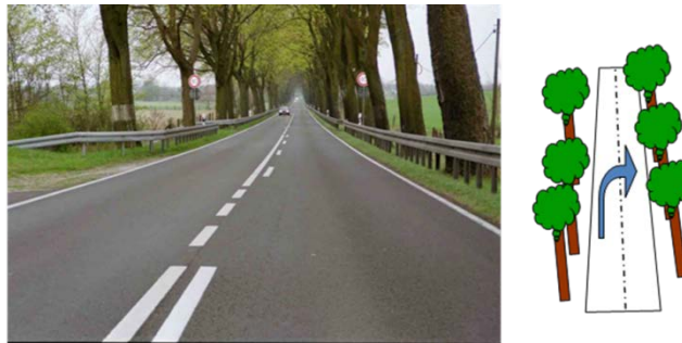
Figure 9. Destabilisation by non-orthogonal impression in an accident spot field-dependent drivers spontaneously swerve and cause accidents [16]
