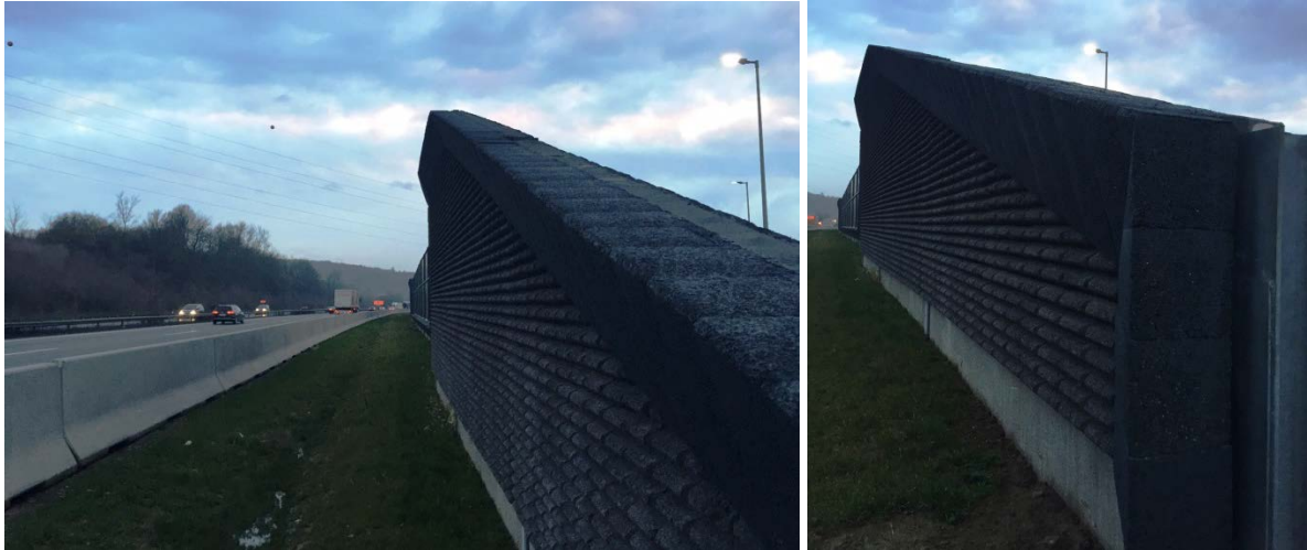
Figure 9/10. Example of a sound-soft element cover, Austria Source: Photograph Ralf Dimberger © DELTA BLOC International GmbH
