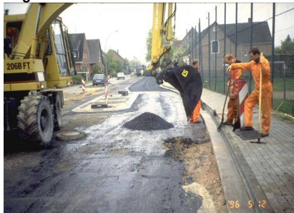
Figure 7. Repair works at the road edge in 1996
