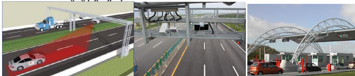
Figure 11. Calm active infrared based tolling
