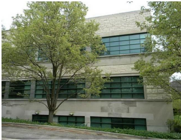
Figure 3 - Overall view of the 1953 building
