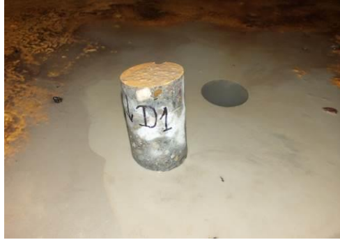
Fig. 17 –Concrete core taken from floor slab
