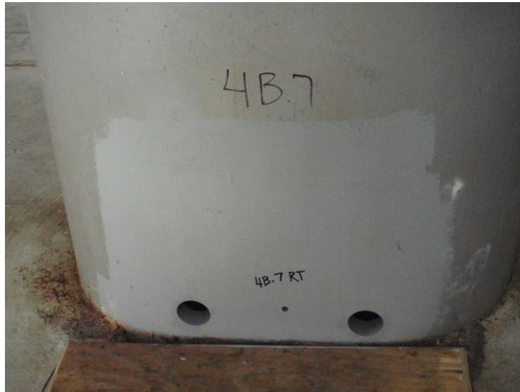
Figure 11. Weld 1 - drilled hole retrofit
