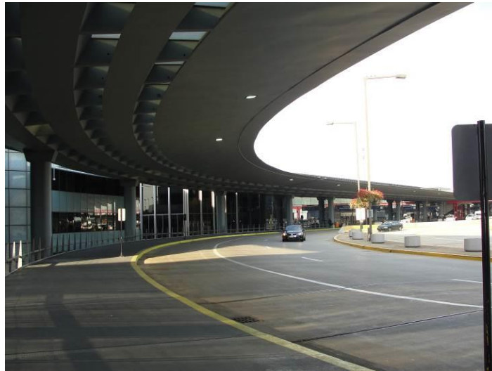
Figure 1. Pedestrian canopy at O'Hare International Airport
