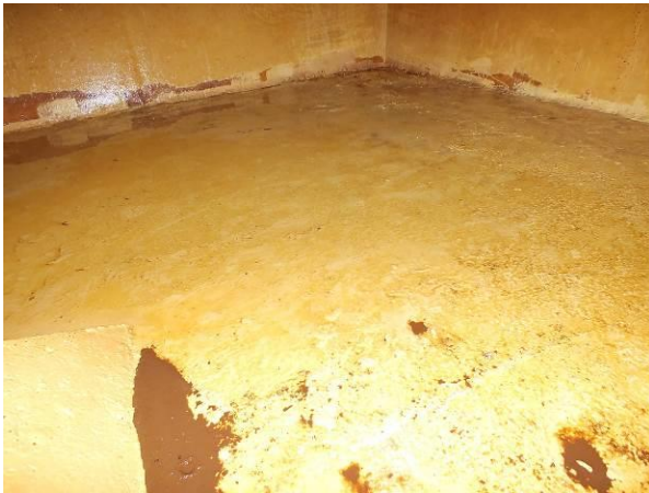
Figure 15 – The appearance of foundation slab
