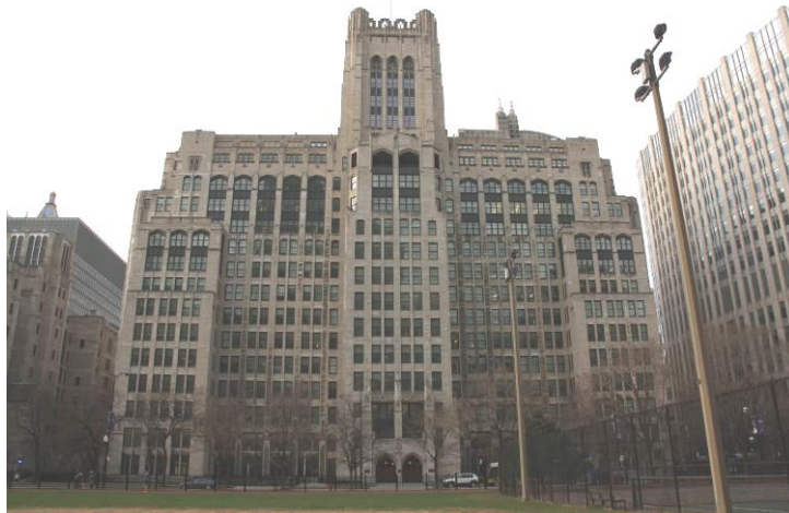
Figure 1 - Overall view of the Montgomery Ward Building
