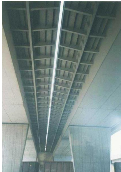
Fig. 3 “Brussels blvd” steel bridge.
