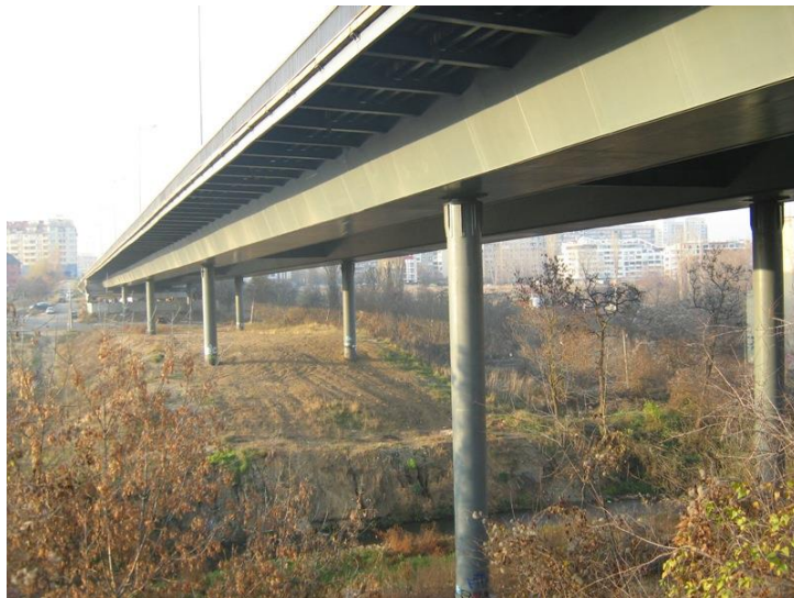
Fig.6 “Vartopa” bridge. (Courtesy of P. Staykov. With permission.)
