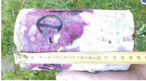
Figure 19 – Measuring of carbonised concrete layer depth – RC wall (10mm)
