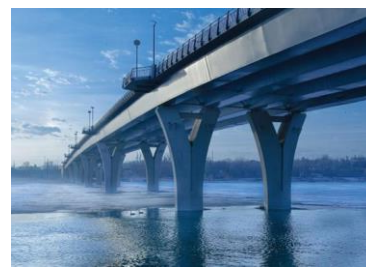
Slika 14 - New Liberty Memorial Bridge, SAD [36]
