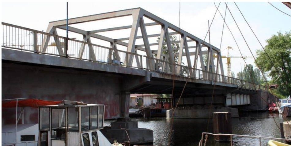
Figure 7 “Varna Lake” movable bridge.
