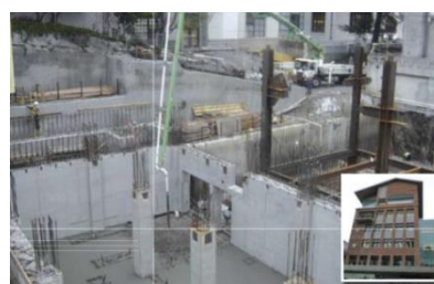
Slika 10 - Izgradnja CITRIS Building, University of California, Berkeley, SAD [32]
