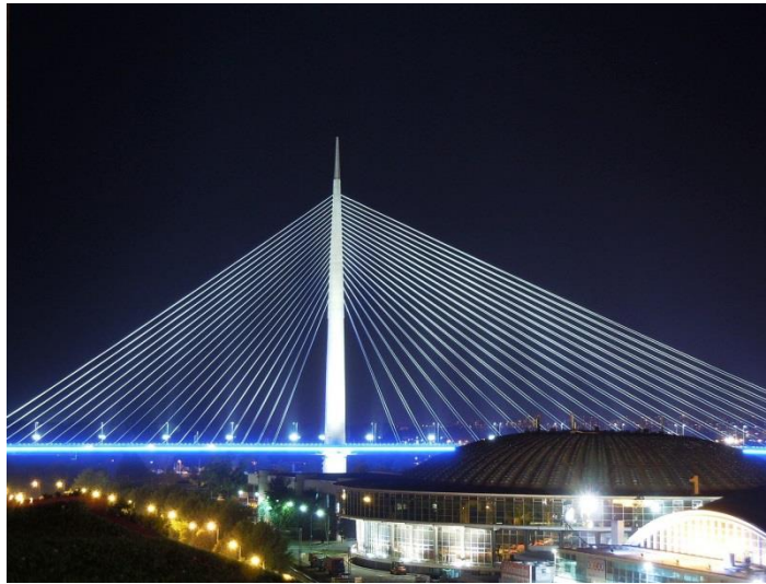
Figure 2 – Side view of Ada Bridge, the new Sava crossing at Belgrade with pylon, cables and girder, [3]
