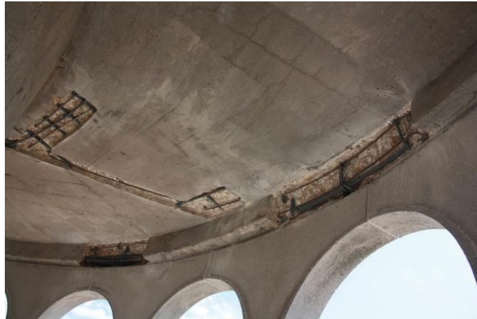
Figure 9 - Repairs in progress on the underside of structural slab
