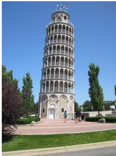
Figure 1 - Overall view of the Leaning Tower in Niles
