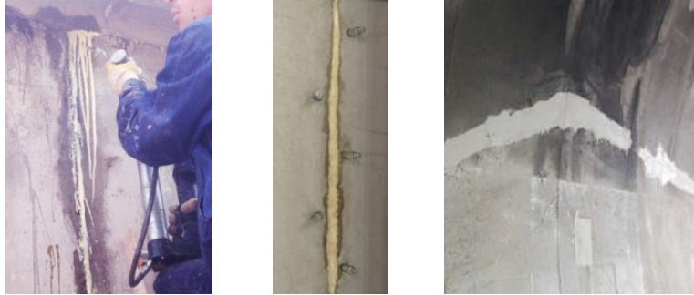
Figure 8 - Injecting a crack
