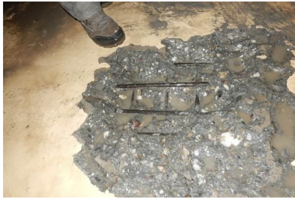
Figure 21 – Upper side of foundation slab, destructive method, reinforcement arrangement
