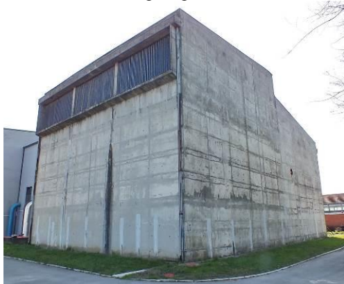
Figure 1 – The appearance of the facility
