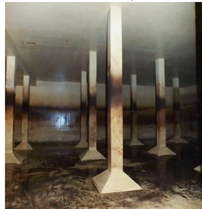
Figure 2 – View of interior of reservoir
