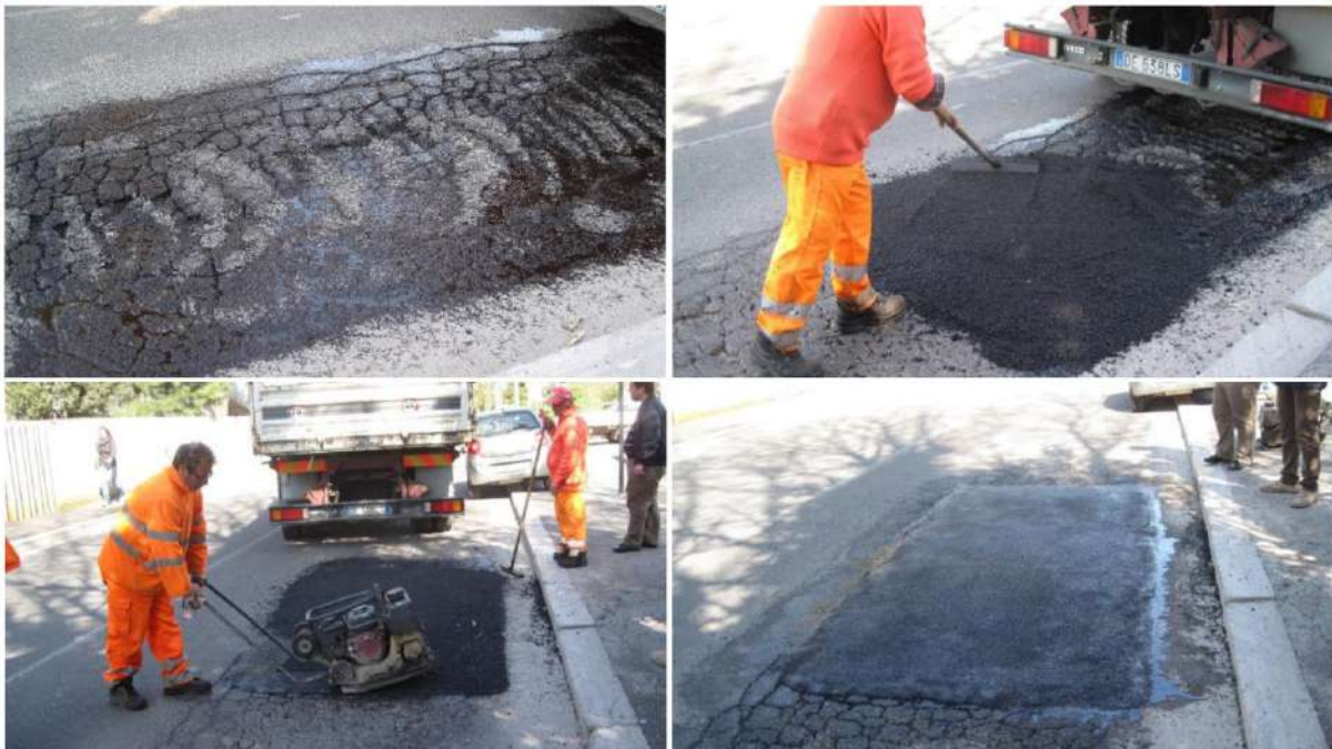
Figure 9. Thin layer overlay, Rome, Italy
