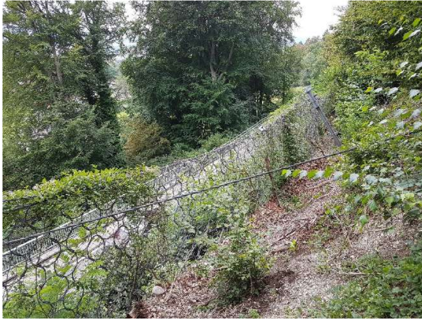
Figure 7. Barrier filled in over time Source: (Gebrugg AG)
